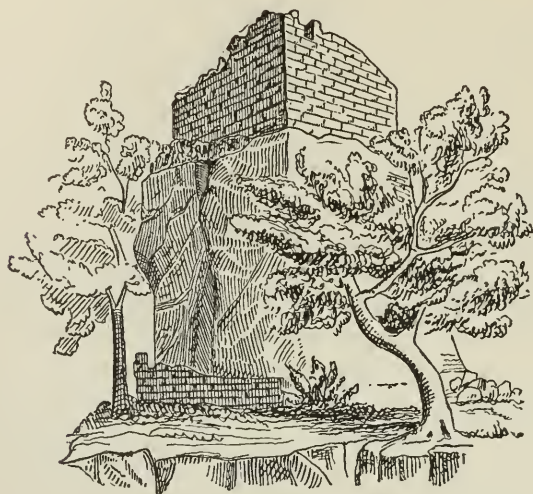
Tower on the McElmo, Colorado.
